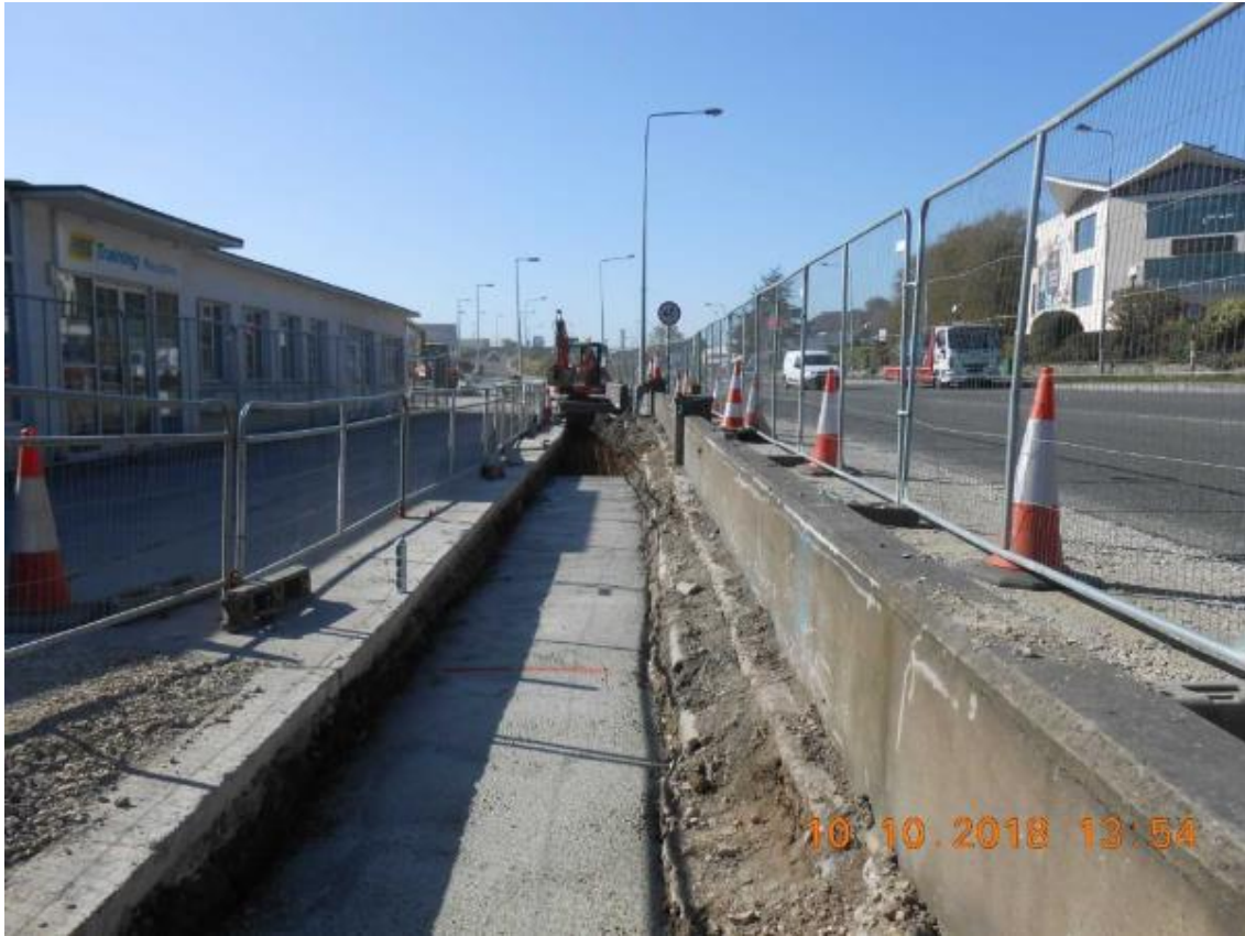
Foundation of new wall at HSS premises.
