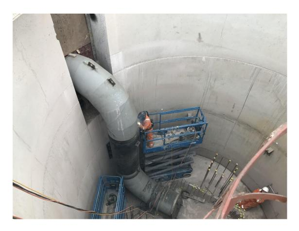
Pipe installation works including pipe welding being progressed in the concrete caisson immediately south of the N25 westbound diverge.
