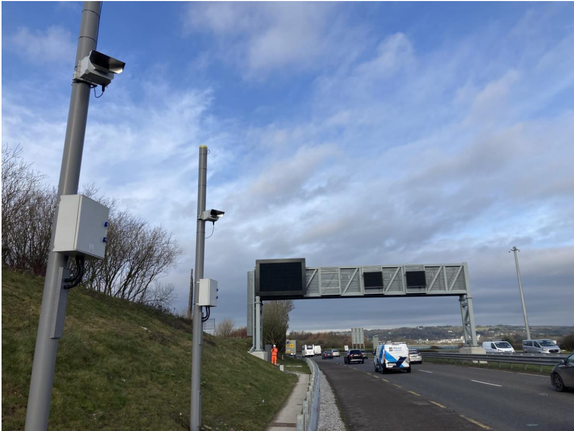
Over-Height Vehicle Detection cameras in place on the N40 northbound approach to the Jack Lynch Tunnel.
