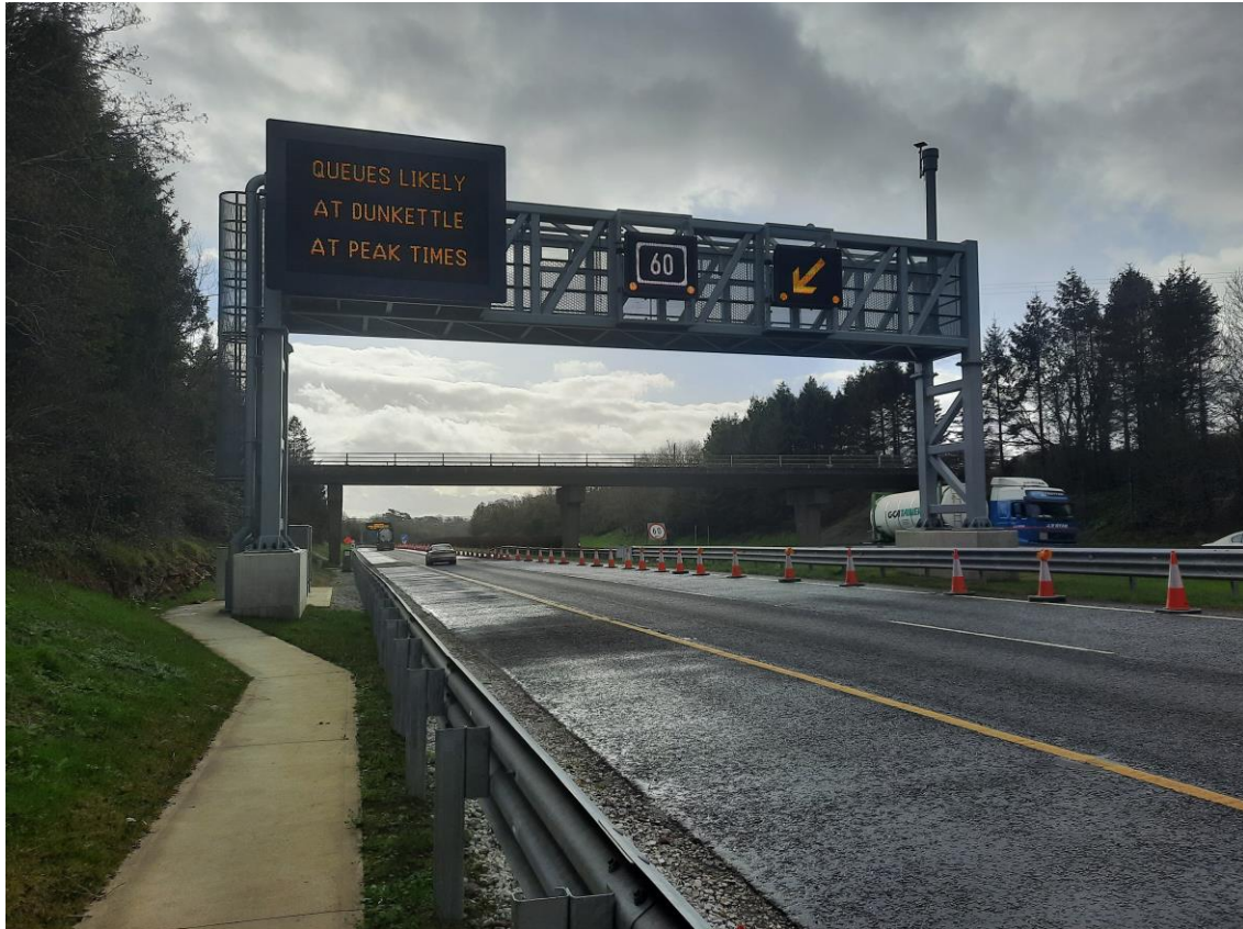
Variable Message Signs (VMS) and Lane Control Signs (LCS) on the M8 southbound approach to the Dunkettle Interchange.
