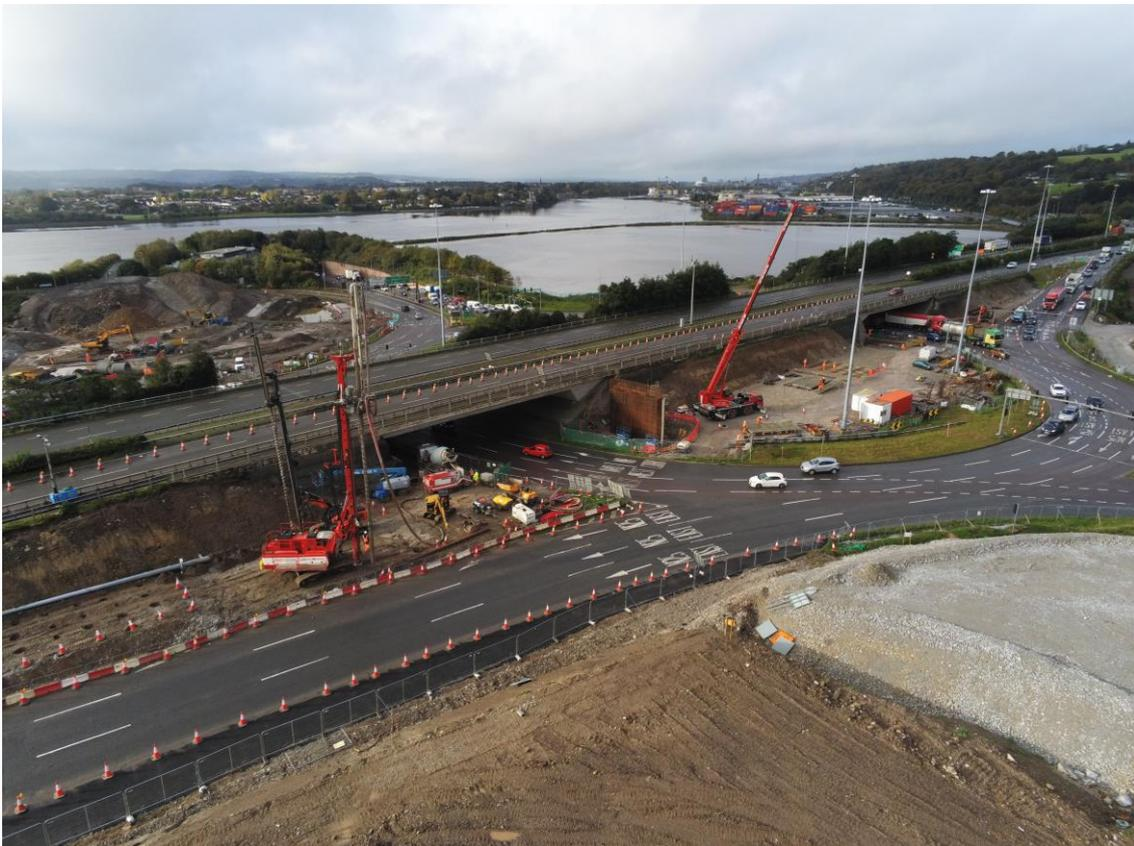
Ongoing piling works for the widening of the existing N25 embankment.
