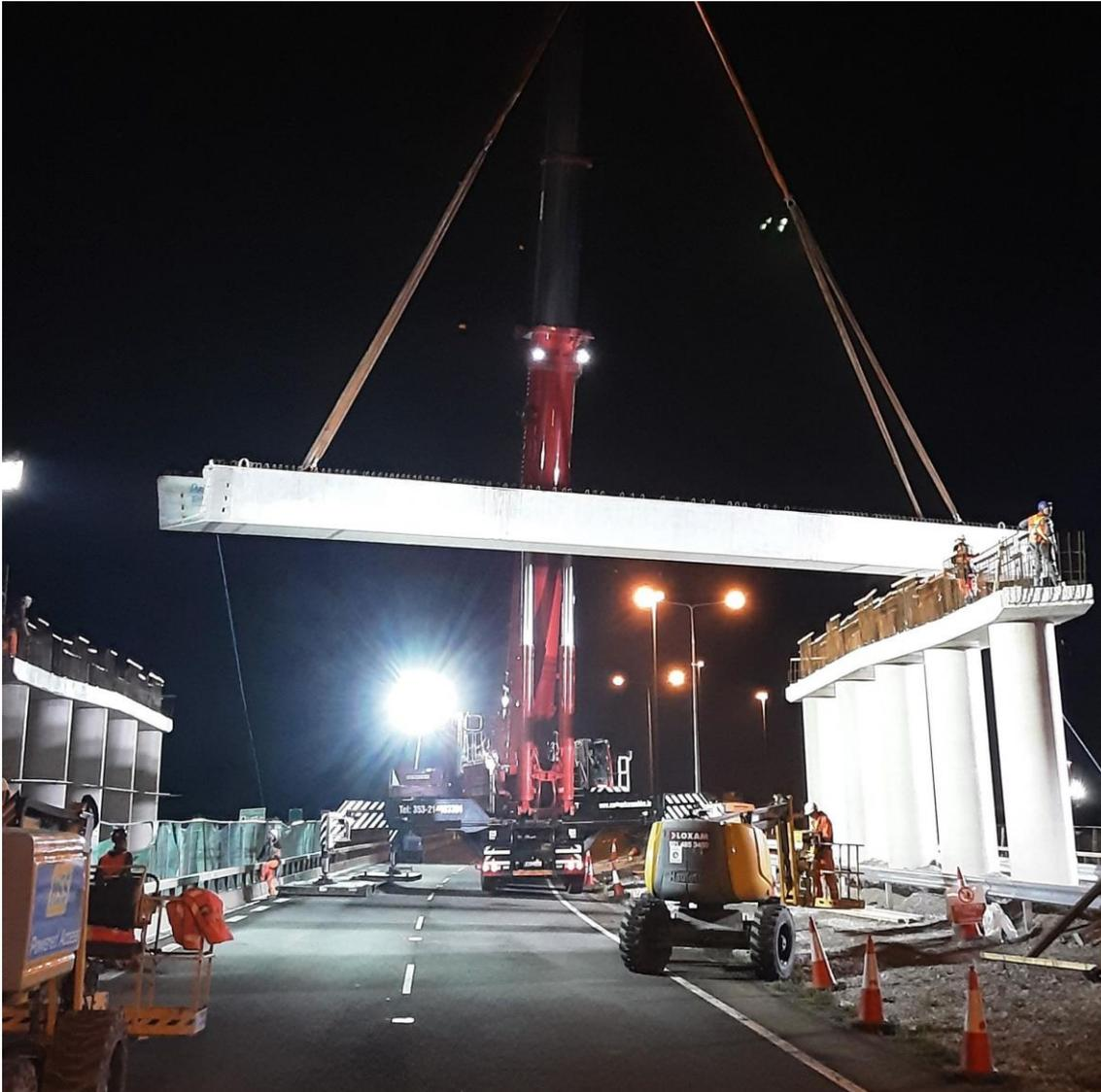
**Installation of beams on Structure ST01 under a night time closure.**
