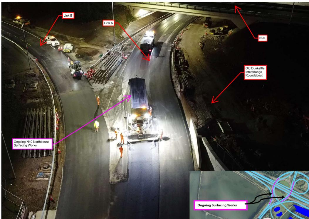
**Surfacing works being undertaken on the N40 North of the Jack Lynch Tunnel under night-time working**
