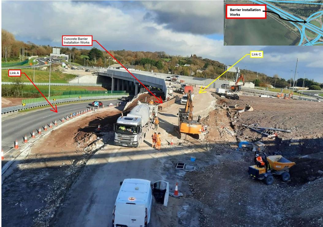
**Works ongoing for the installation of the new concrete safety barrier between Link A and Link C in the vicinity of the old Dunkettle Interchange Roundabout**
